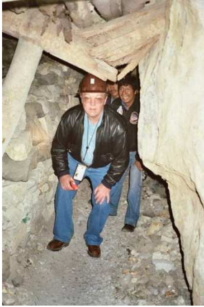
Jhonny Horozco follows Stuart as they approach a broken beam
